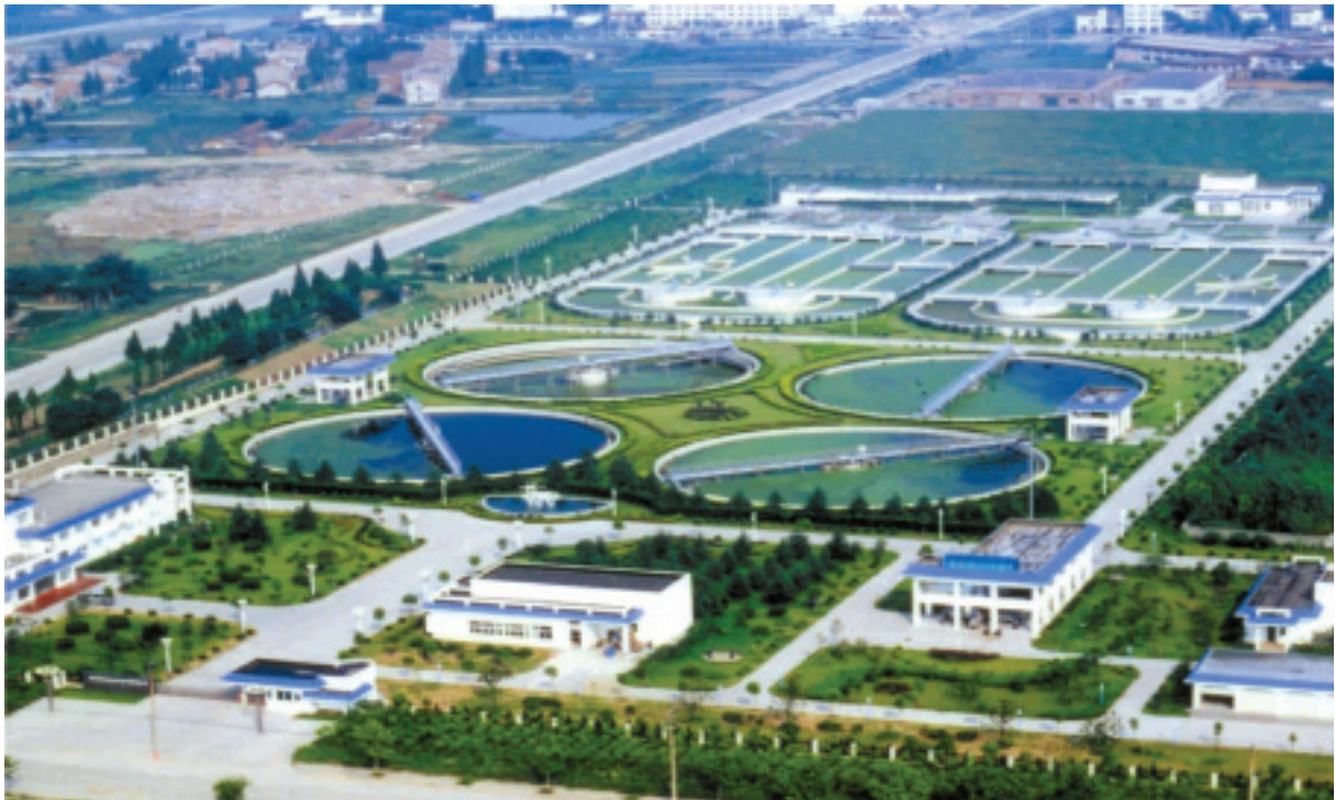
Hongguang sewage treatment plant of Jingzhou Water Environmental Protection Co., Ltd.
