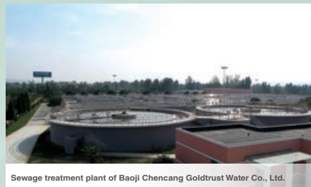
Sewage treatment plant of Baoji Chencang Goldtrust Water Co., Ltd.
