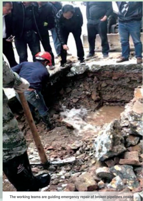
The working teams are guiding emergency repair of broken pipelines onsite
