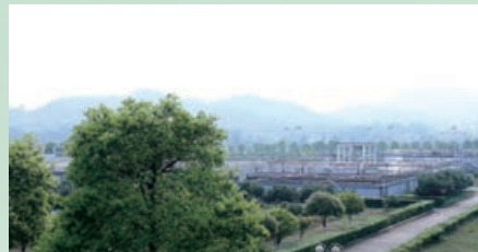
Sewage treatment plant of Fenyi Environmental Co. Ltd.
