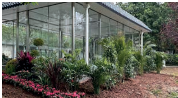
Restoring greenery after the completion of the sun-lit glass machine room for the direct drinking water business
