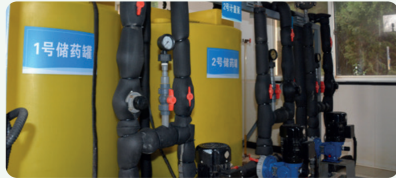
Implement freeze prevention and insulation measures for equipment and pipelines
